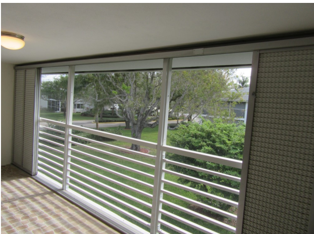
Non rated sun shutters on the east patio
