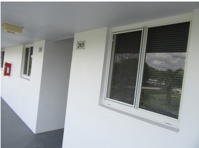
West side windows are Miami Dade impact rated as determined by etching on glass
