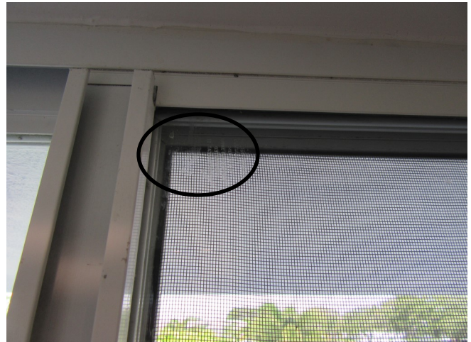
West side windows are Miami Dade impact rated as determined by etching on glass
