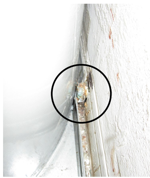
The pan under the hot water heater has been replaced. Where the drain line connects it is not properly secured and sealed. If the heater were to leak into the pan the pan would over flow when reaching approximately 1/2" of water.
