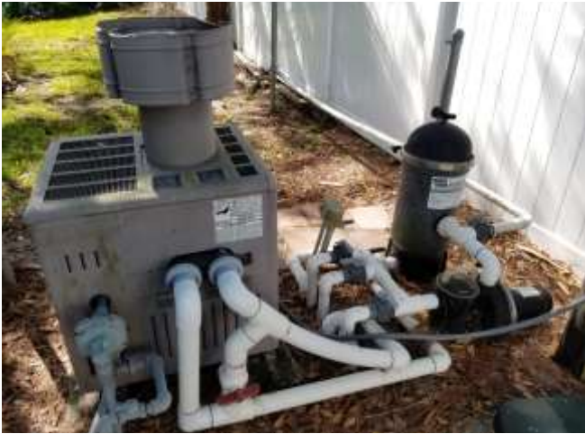
The pools finish was good, the light was lit and a water fall function was noted to work. The pool motor and filter appeared older and possibly original but no defect was noted. The pools gas heater did not start.
