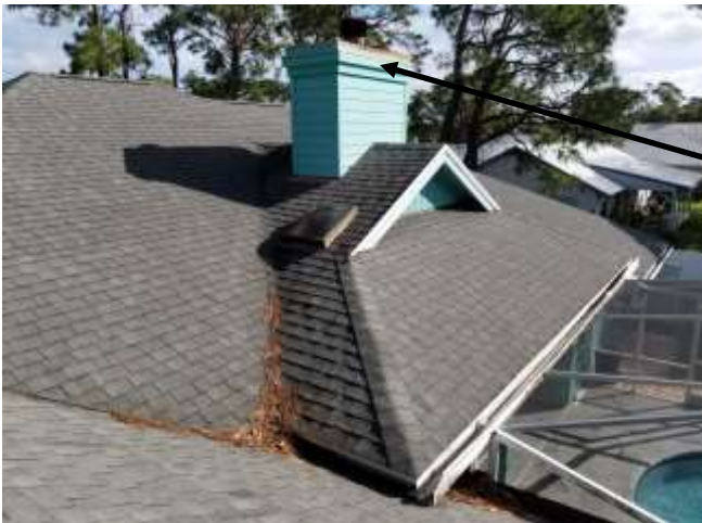
The chimney cap was sound and does not leak is but is rusting on its top. Properly cleaning, treating and painting will extend it's serviceable life.
