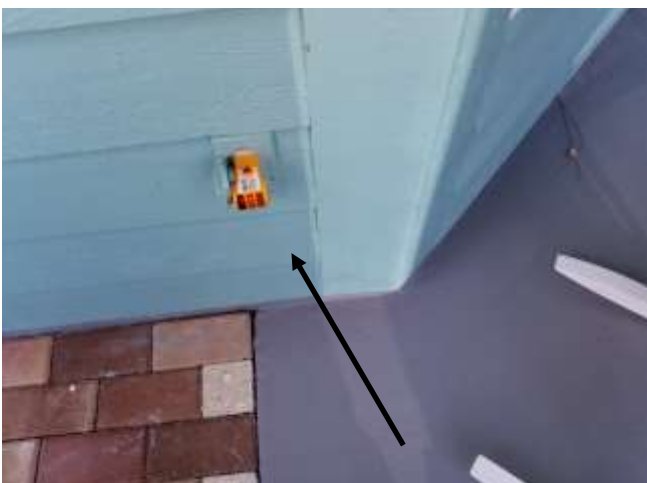
The exterior and garage outlets are not GFCI protected and should be since 1975. *There is a GFCI type outlet on the patio by the family room door which did not trip off when tested. *The outlets on the exterior front and east side have their black and white wires connected in reverse. The outlet on the patios master bedroom wall is loosely secured to the electric box.
