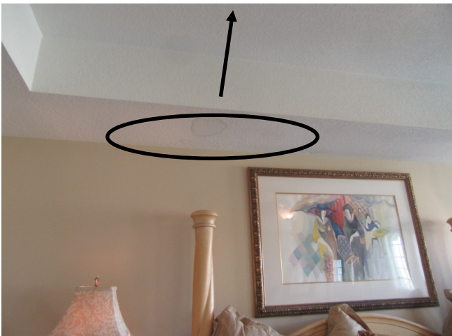
In the third floor master bedroom ceiling above the bed left side when facing it there is a water stain. In the attic above this area there is some staining on the fire rated sheetrock on the wall between the two units. It is thought there is a leak at the chimney of the neighboring unit which is in the same location. Due to the roof elevation and location the roof could not be physically and visually inspected.
