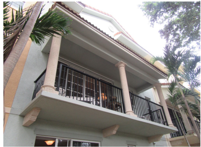
Miami-Dade impact rated windows and doors on the second and third floors and corrugated Miami Dade rated shutters for the first floor openings stored in the garage.
