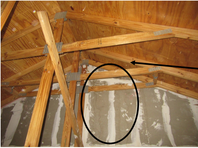
In the third floor master bedroom ceiling above the bed left side when facing it there is a water stain. In the attic above this area there is some staining on the fire rated sheetrock on the wall between the two units. It is thought there is a leak at the chimney of the neighboring unit which is in the same location. Due to the roof elevation and location the roof could not be physically and visually inspected.
