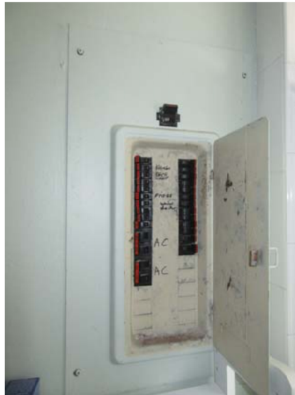
Federal Pacific brand electric panel with a 150 amp main breaker located in the hall bathroom. No tampering was noted.
