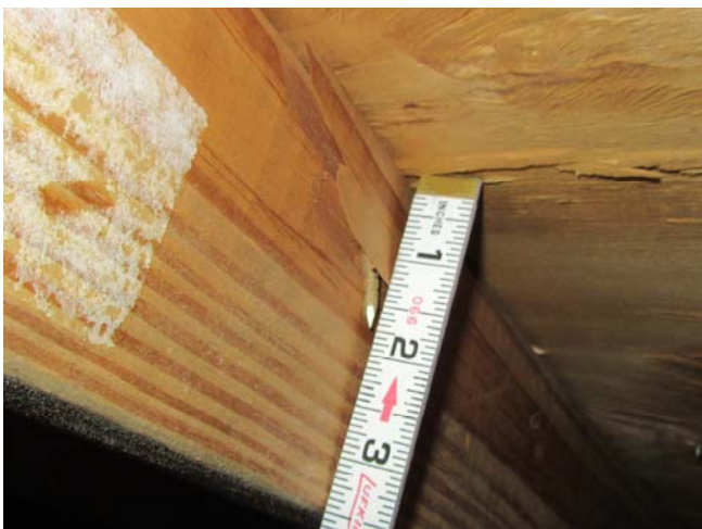
Roof nailing pattern of 8pn nails installed 6" oc center in the field and 6" oc center on the edge is determined with the use of a Zircon MT6 metal detector.
