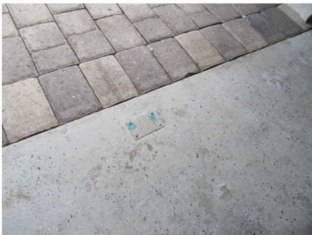
Wind Pressure resistant garage door attachment was noted
