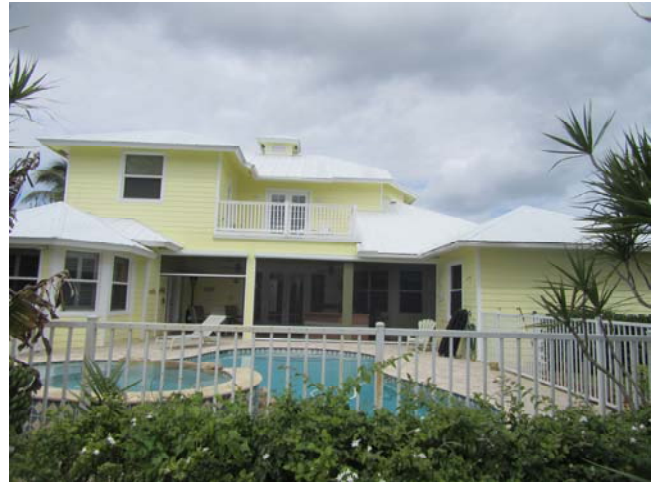
Roof permitted original
