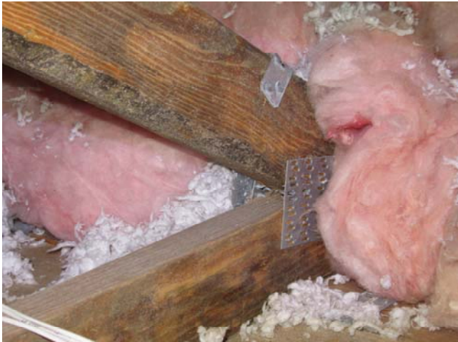
Single wrapped metal straps wrapping the top of the truss used to secure the roof rafters to the CBS walls.
