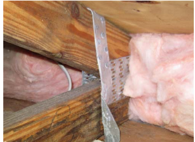
Single wrapped metal straps wrapping the top of the truss used to secure the roof rafters to the CBS walls.
