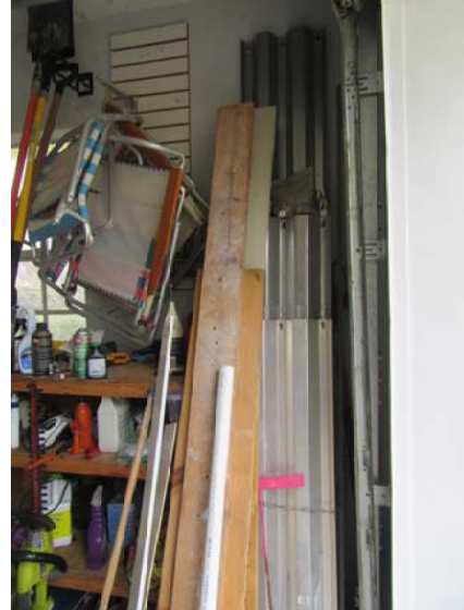
Corrugated shutters are located in the garage for all first floor openings.
