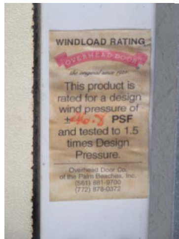
Wind Pressure resistant garage door attachment was noted
